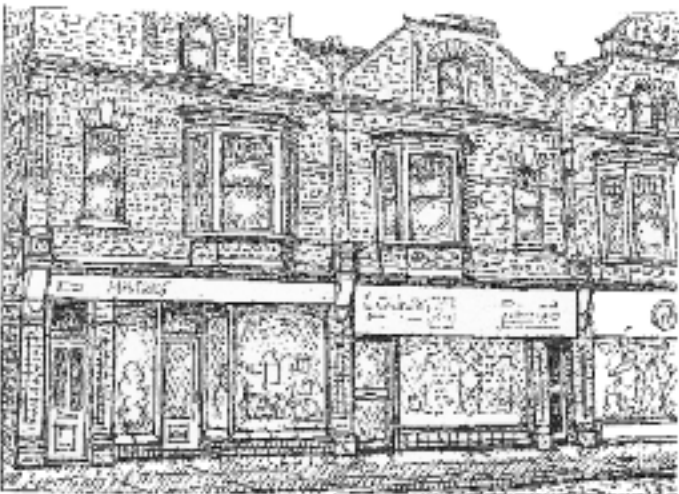
FIG.9. The front (probably of early 20th century date) on the far left is contemporary with the building. The door to its left hand side leads to a stair to the upper levels. The shop entry is via an off-centre in-go placed to catch the eye of passers-by. The signboard is of the traditional shallow depth, the window display 'reading' as the shop's main advertisement. By contrast the adjacent deep modern signboard competes visually with the window below and is too large for the building. It conceals the original shallow depth fascia which could easily be exposed to bring back an element of design quality to the overall composition.
