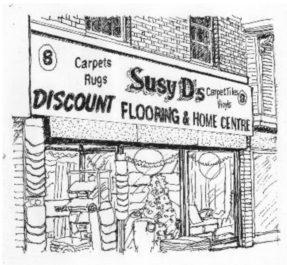
FIG.27. An example of signage in common use but unacceptable in conservation areas. The signboard is too deep for its location on a traditional brick building. The metal box containing an external roller shutter is crudely exposed below the signboard, adding to the latter's effect of depth. A number of different type fonts are employed on the signboard and this together with their detailed relationship to one another, gives visually competing messages. One main message should stand out.
