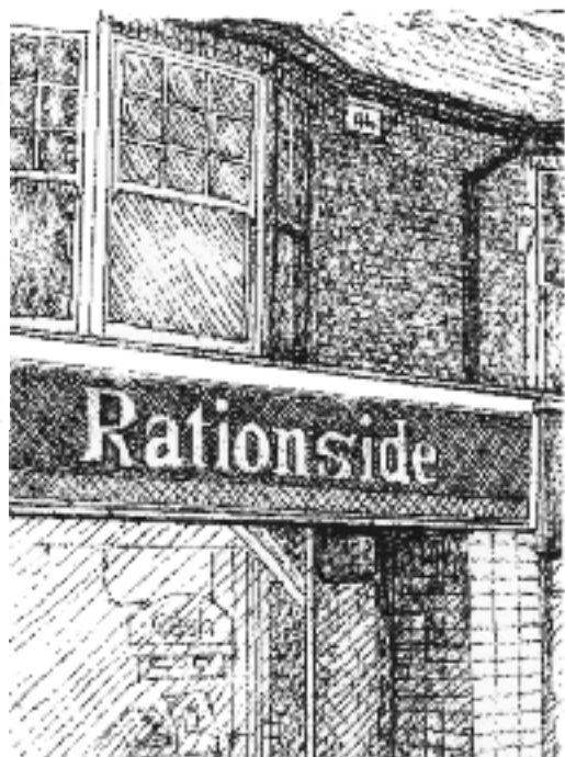
FIG. 12. A shop front replacing a previous one that was related architecturally to the first floor façade. The deep, flat, box-fascia is over scaled for its location. The single paned shop window is framed in narrow flat strips of stainless steel and the flat sides of the pier on the right are clad in shiny glazed tiles. These features are not acceptable as they detract from the character of the building.
